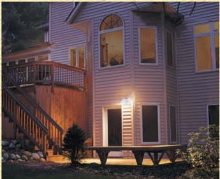
Motion Activated Security Lighting
